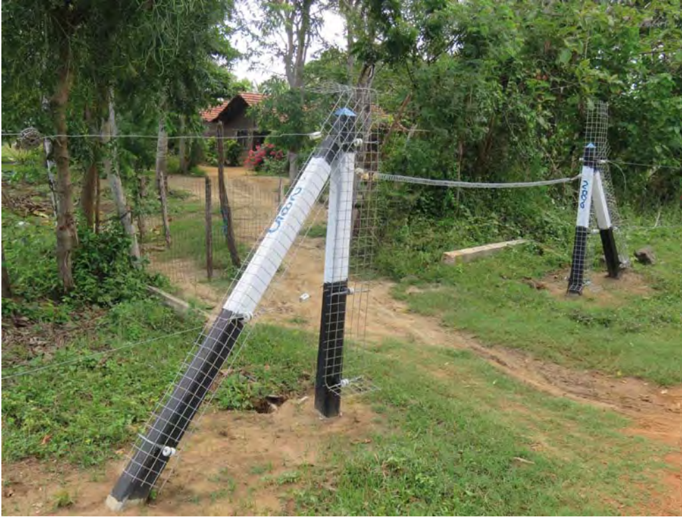
Photograph 19 Gate with gate-spring unit in place. Note flanking posts supported by jack posts. Tammannawa, Hambantota District, Sri Lanka.
