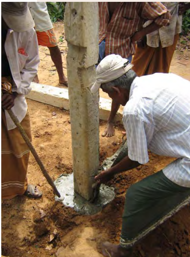
Photograph 18 Concreting a fence post in place. Mudaliyarkulam, Trincomalee District, Sri Lanka.
