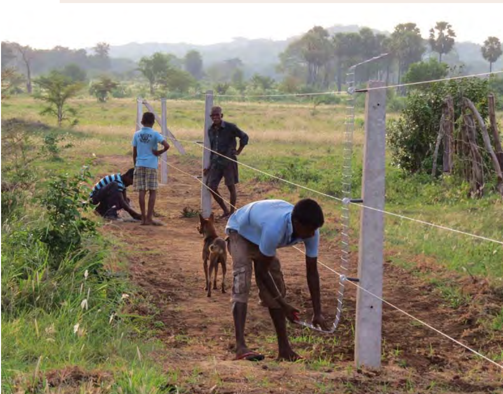
Photograph 22 Installing GI mesh fence post guards. Mudaliyarkulam, Trincomalee District, Sri Lanka.
