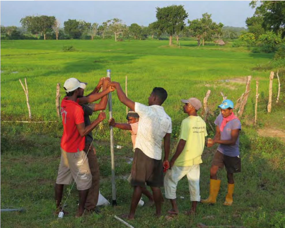
Photograph 31 Supporting corner post with a guy wire. Rotawala, Hambantota District, Sri Lanka.
