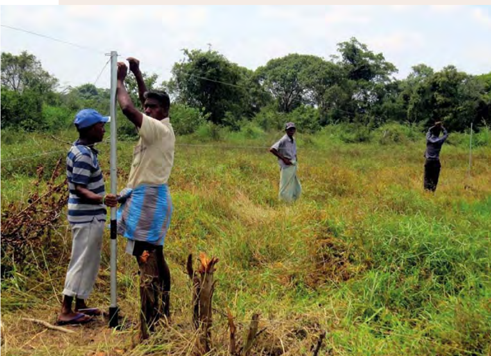
Photograph 32 Pulling the wire. Veppankulam, Trincomalee District, Sri Lanka.
