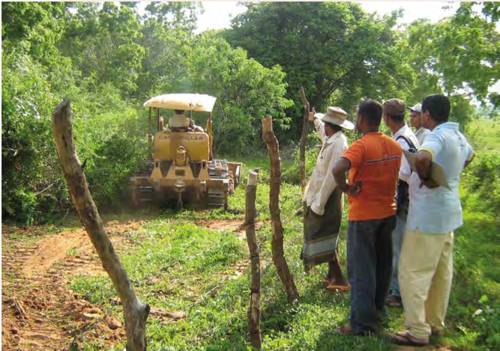
Photograph 11 Clearing the fence line. Bundala, Hambantota District, Sri Lanka.
