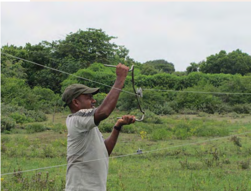
Photograph 21 Adjusting wire tension with the wire tightener handle. Bundala, Hambantota District, Sri Lanka.
