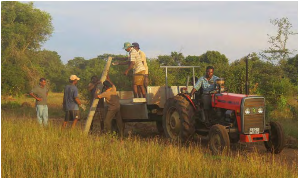
Photograph 17 Unloading the fence posts along the fence line. Panmedawachchiya, Trincomalee District, Sri Lanka
