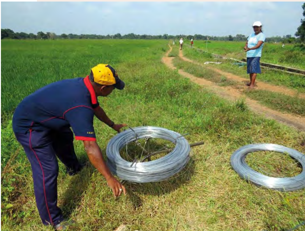
Photograph 20 Dispensing wire with a wire dispenser. Veppankulam, Trincomalee District, Sri Lanka.
