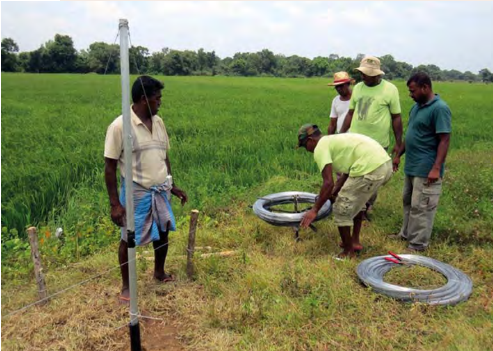
Photograph 33 Dispensing wire with a wire dispenser. Veppankulam, Trincomalee District, Sri Lanka.
